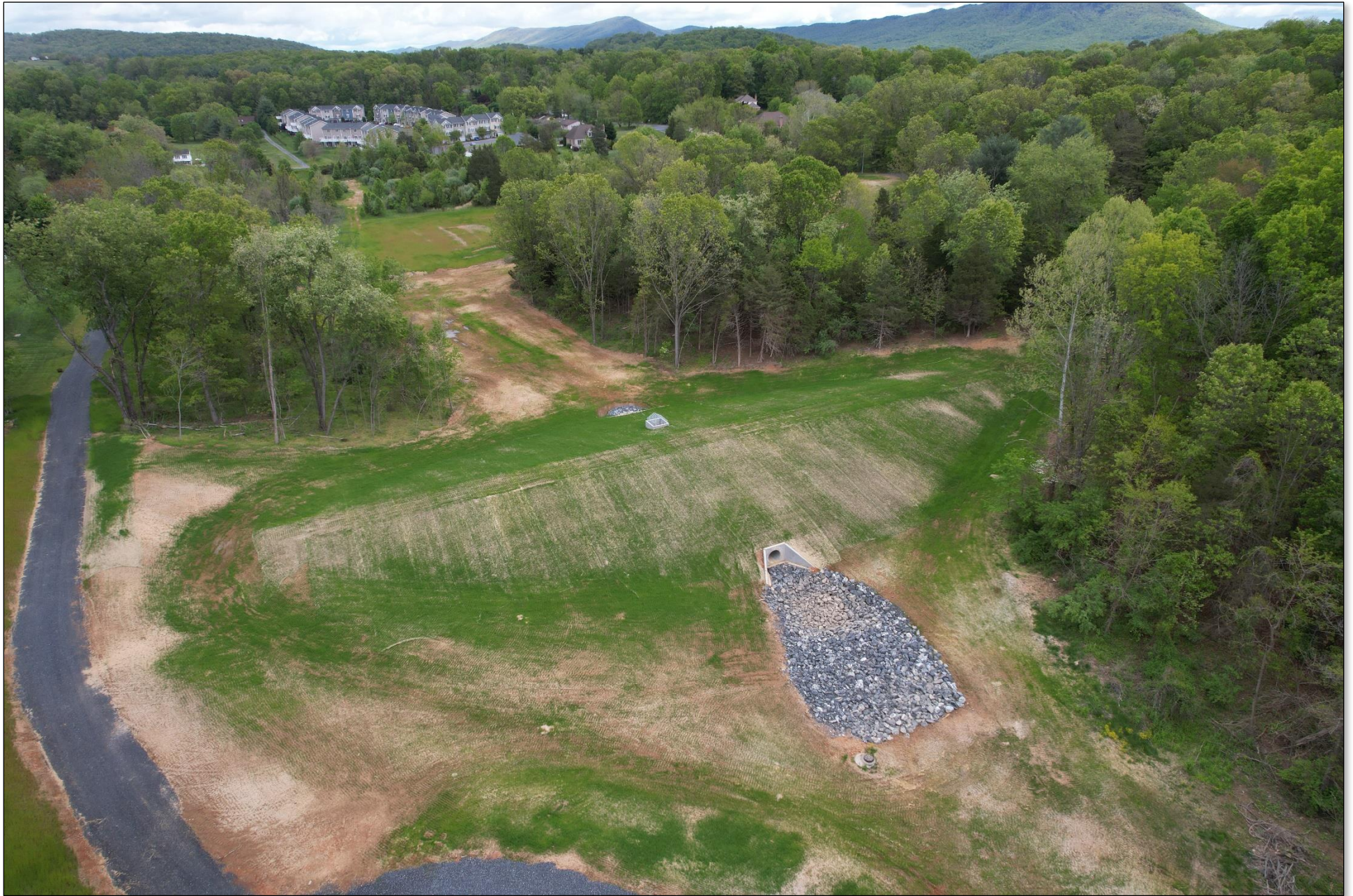
Completed embankment and plunge pool
