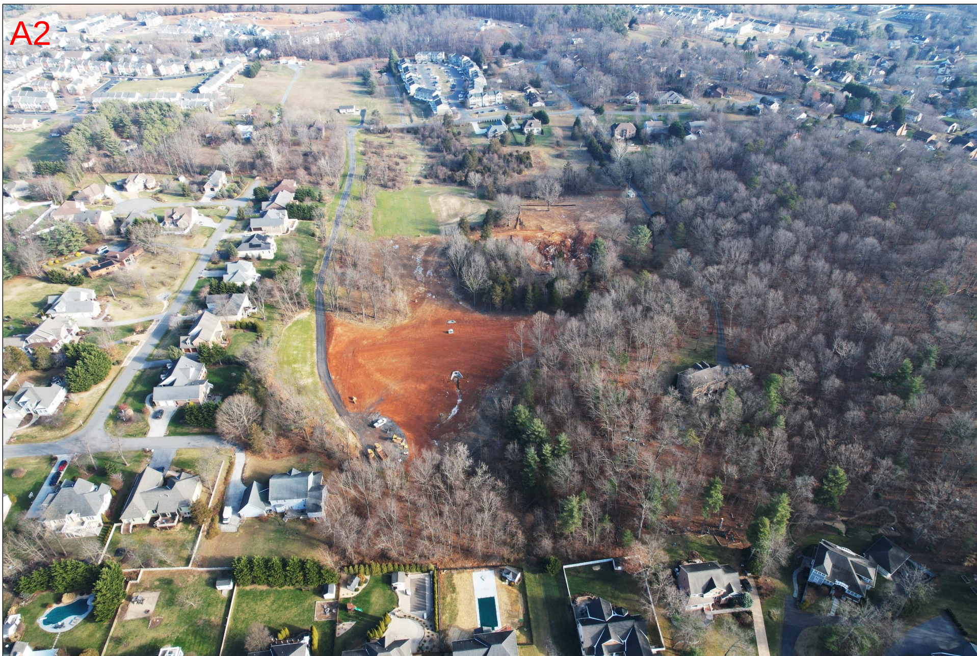
Aerial photo of project site looking northeast
