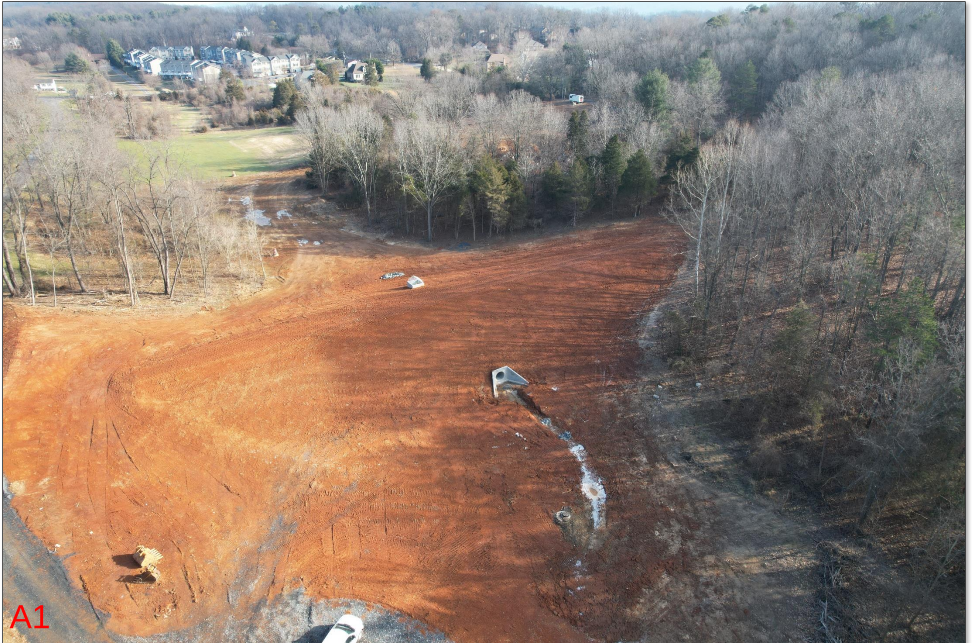
Aerial photo of completed embankment
