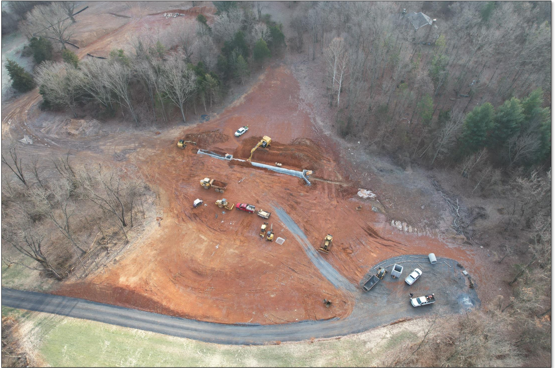
Aerial photo of embankment construction
