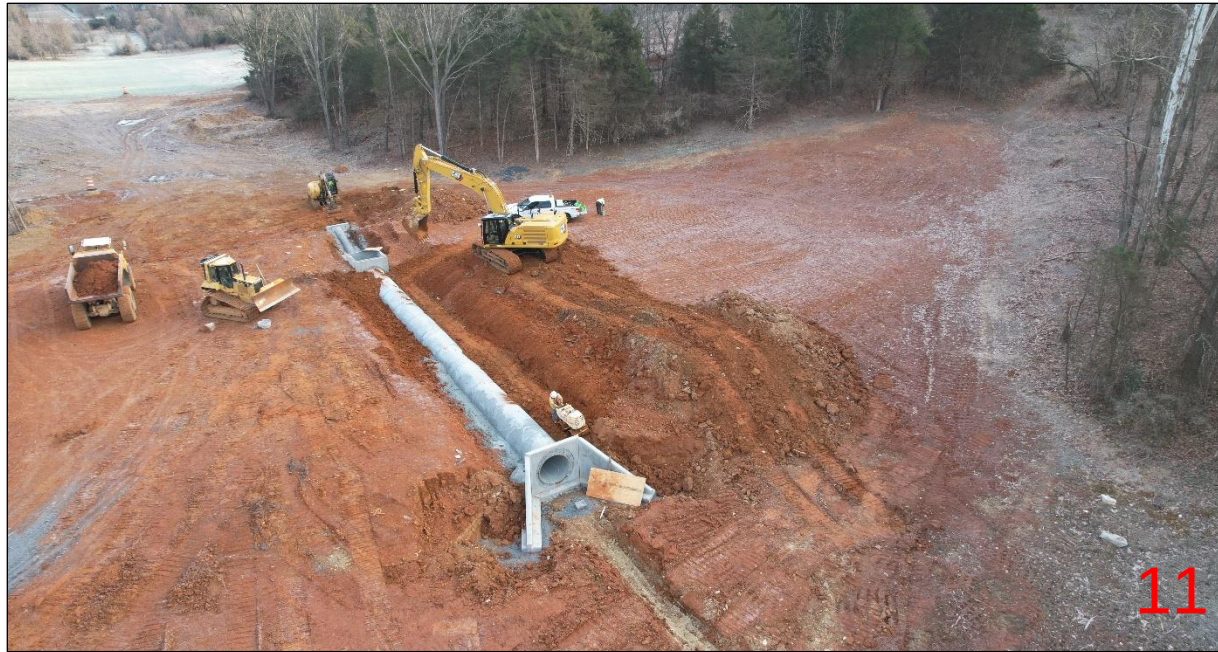
Installation of concrete storm pipes and outlet structure
