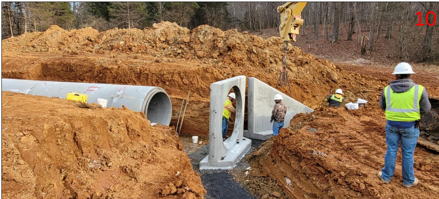
Installation of concrete storm pipes and outlet structure
