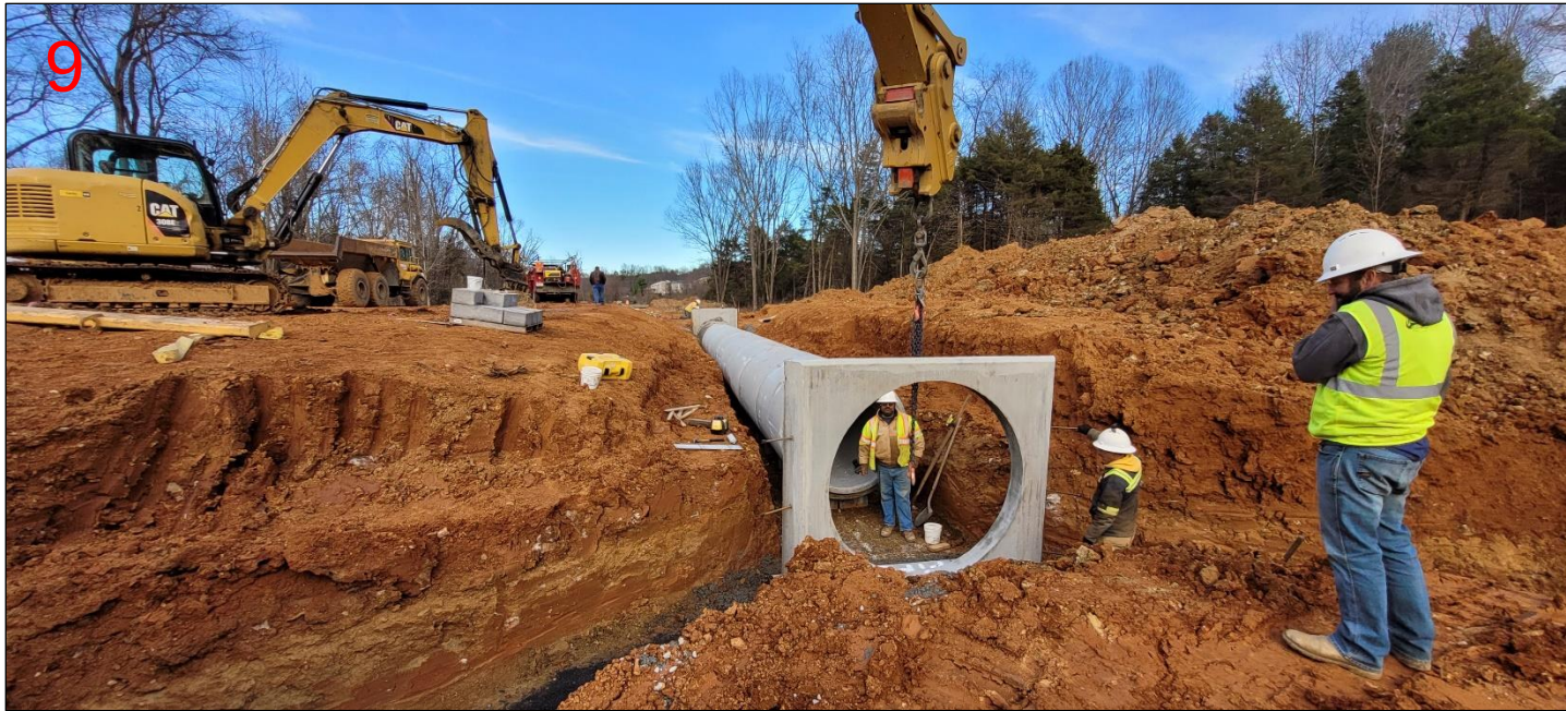
Installation of concrete storm pipes and outlet structure
