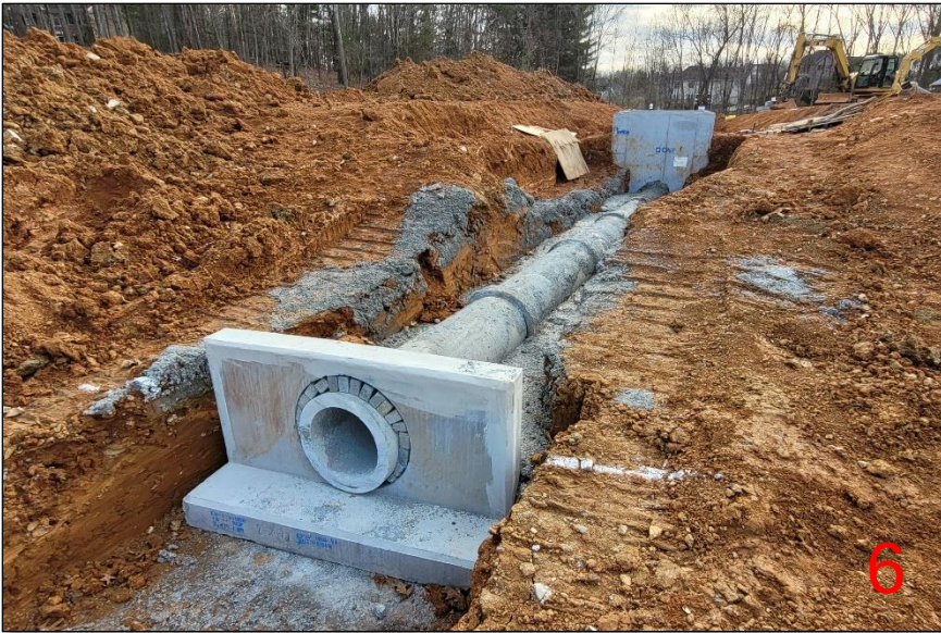
Installation of concrete storm pipes and outlet structure
