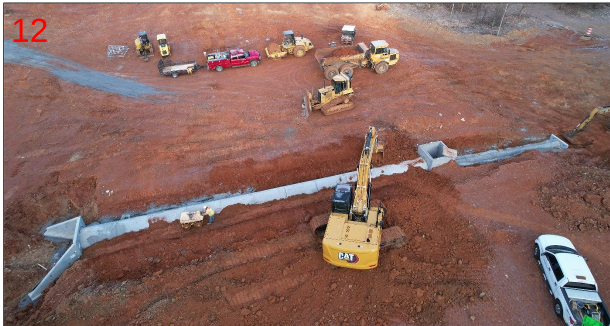
Installation of concrete storm pipes and outlet structure
