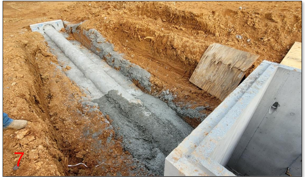
Installation of concrete storm pipes and outlet structure
