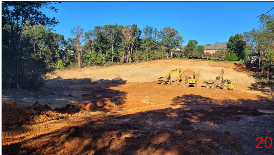
Excavation for embankment cutoff trench
