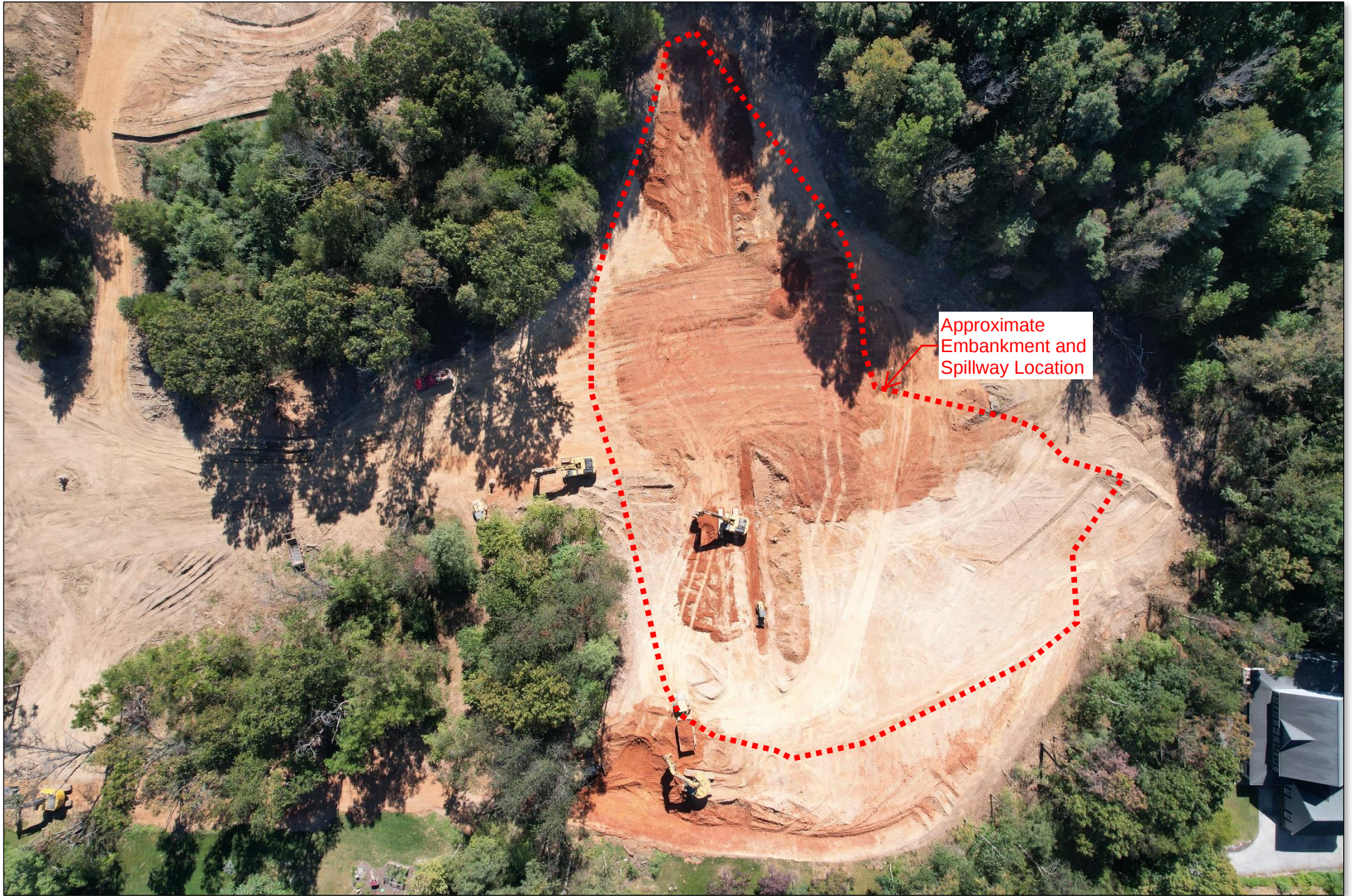
Aerial photo of embankment construction
