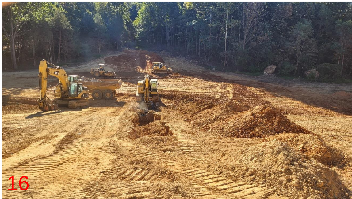
Lower basin and excavation for embankment cutoff trench
