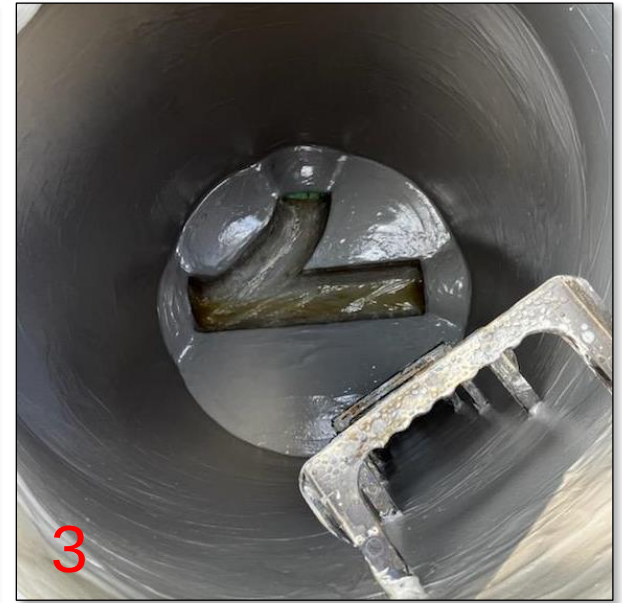
Sanitary sewer manhole rehabilitation (above) and upper basin graded and seeded (below)
