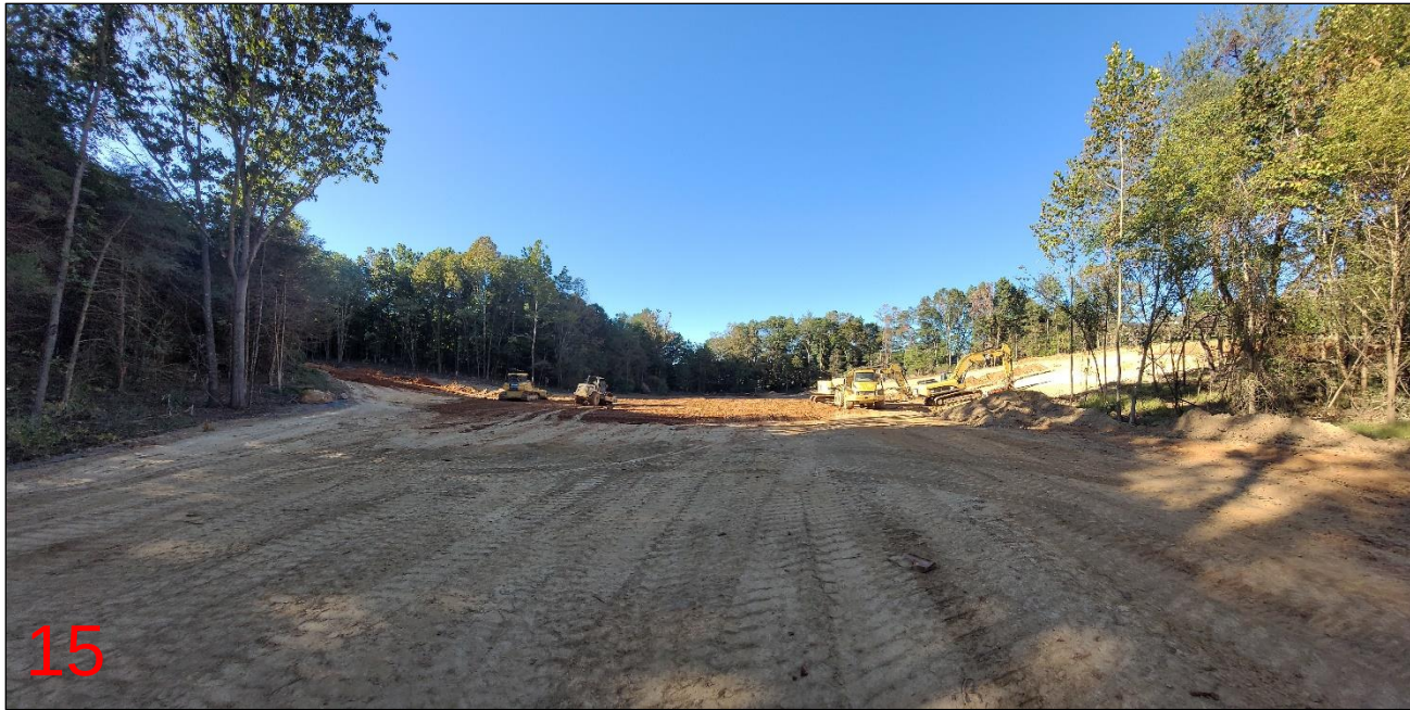
Lower basin and excavation for embankment cutoff trench
