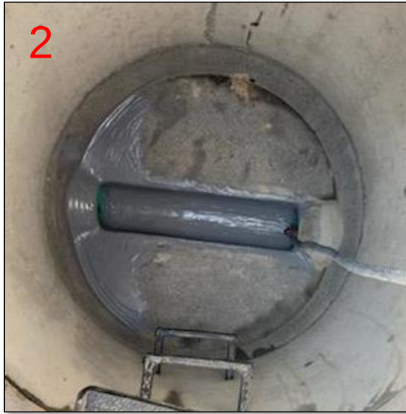
Sanitary sewer manhole rehabilitation (above) and upper basin graded and seeded (below)
