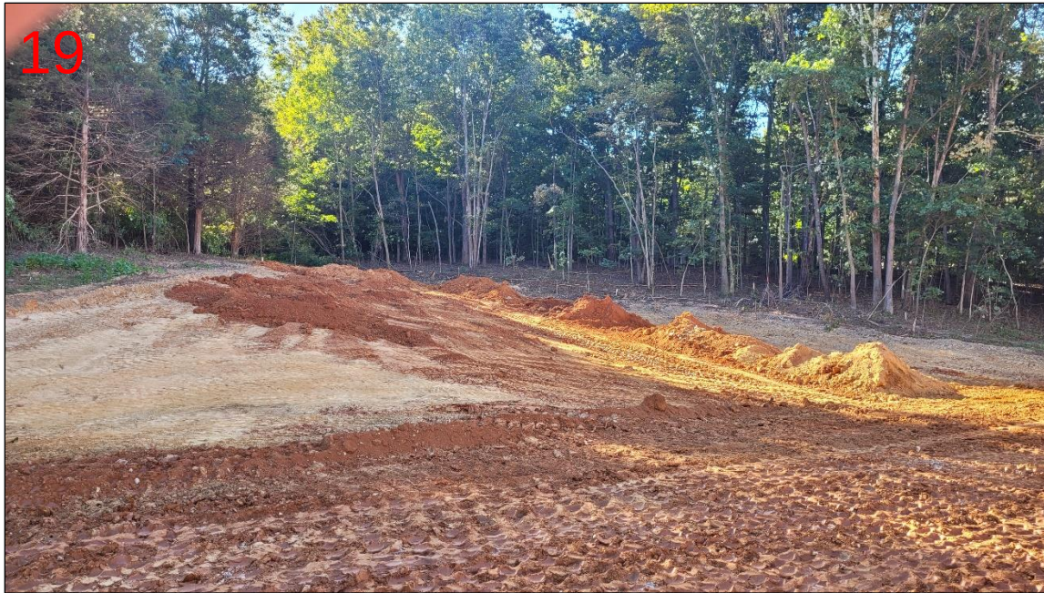
Excavation for embankment cutoff trench
