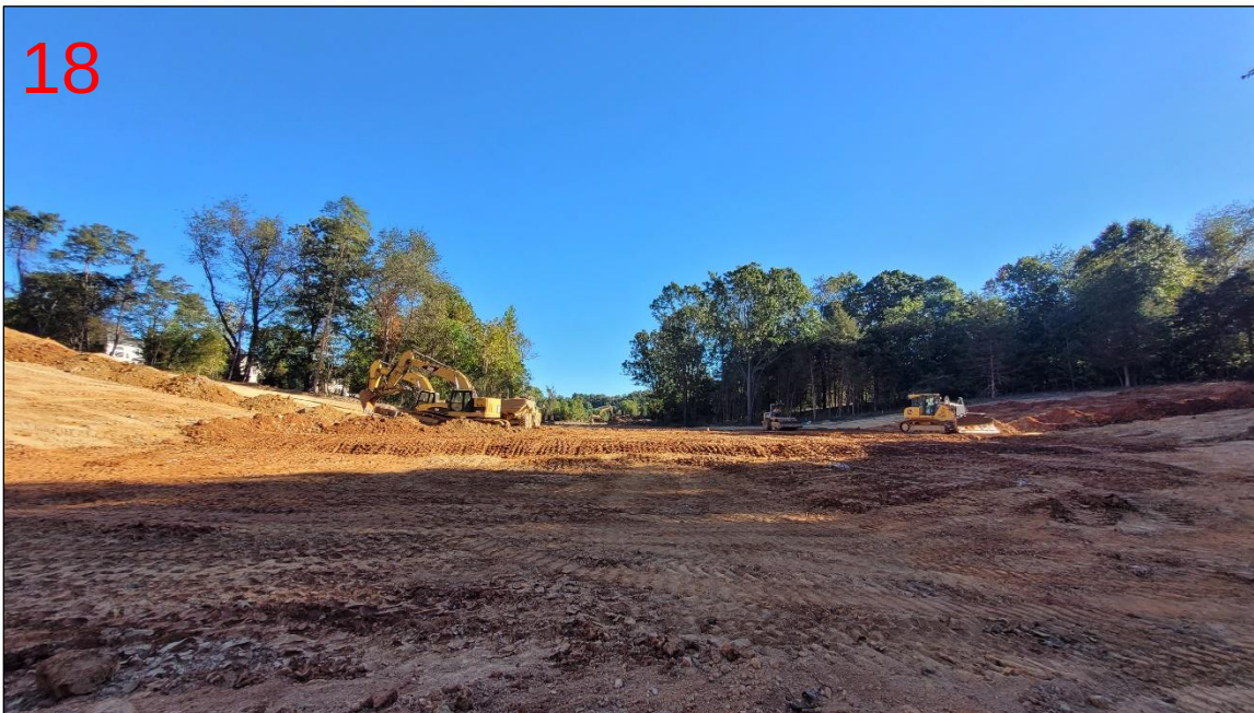
Excavation for embankment cutoff trench
