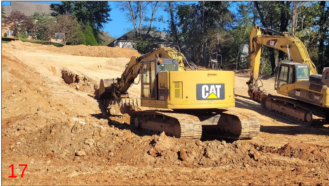
Excavation for embankment cutoff trench
