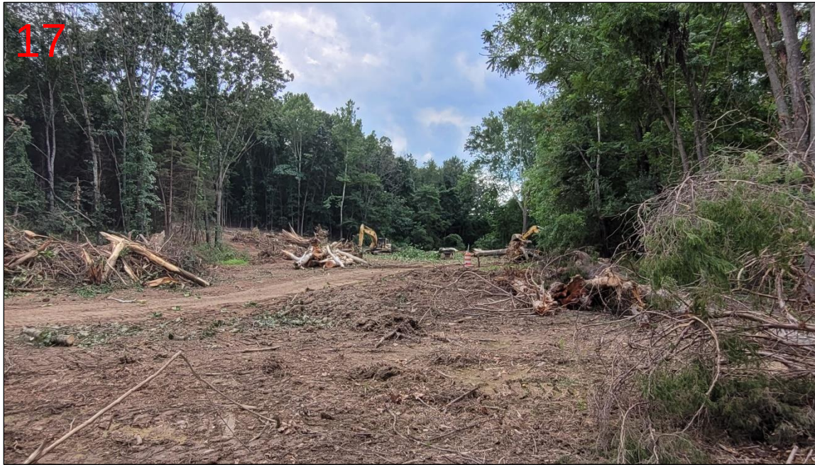
Site clearing and grubbing progress
