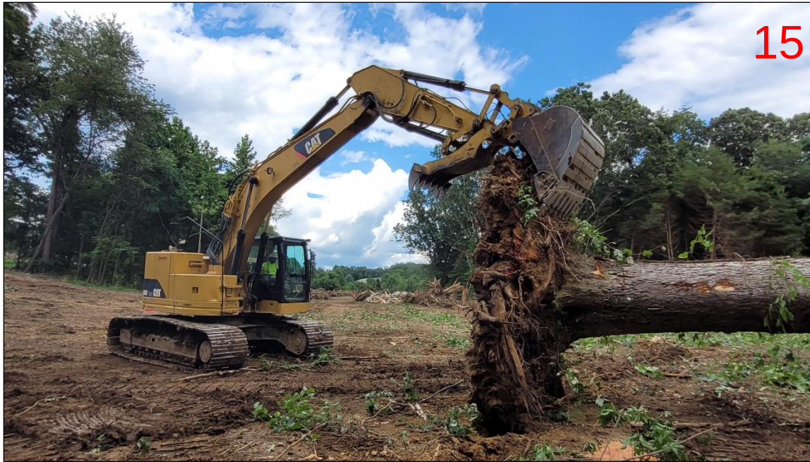
Site clearing and grubbing progress
