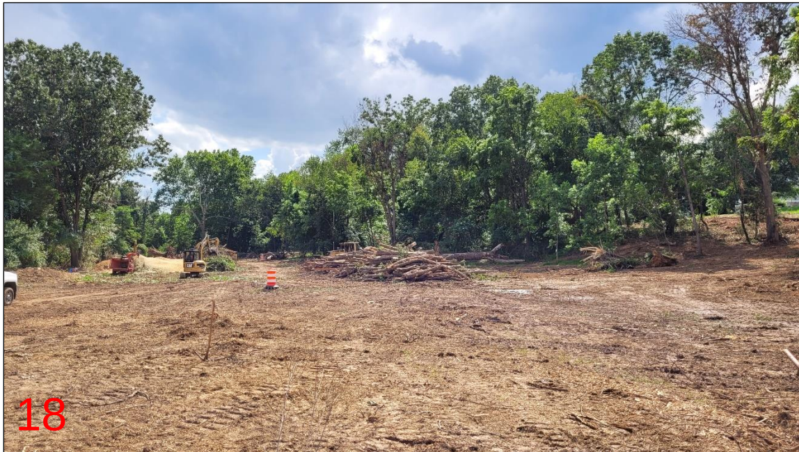
Site clearing and grubbing progress
