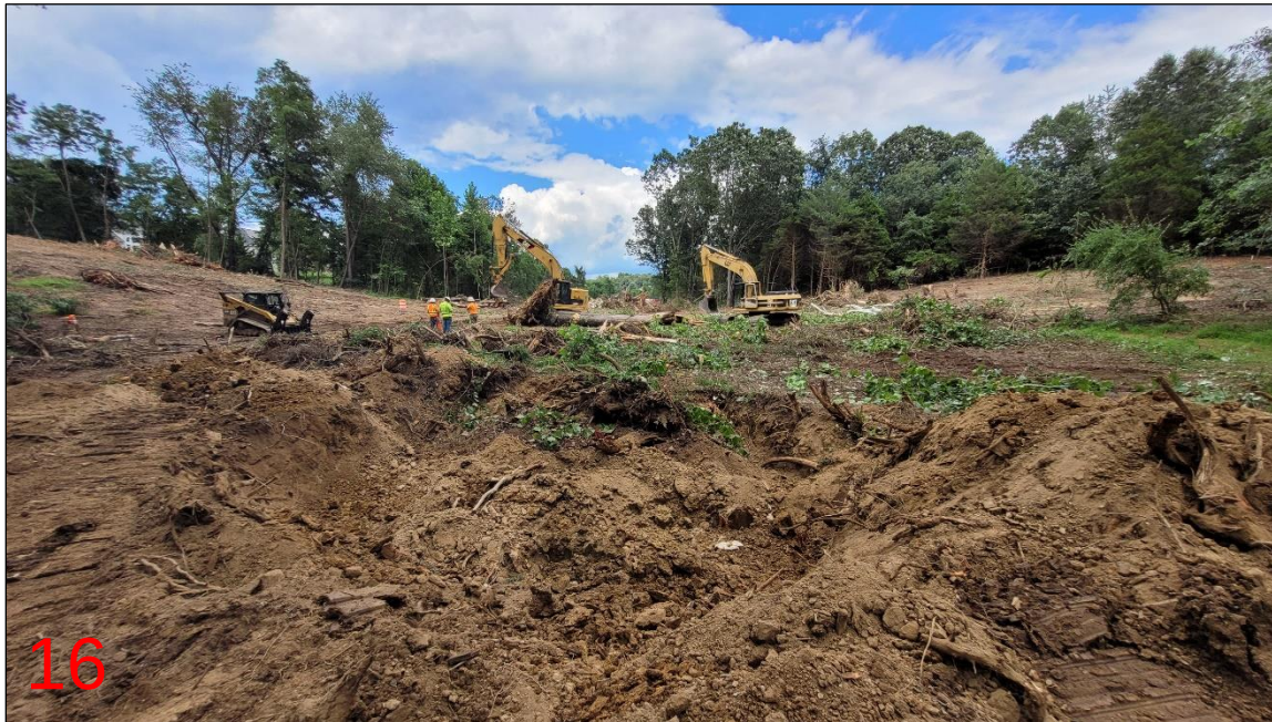
Site clearing and grubbing progress
