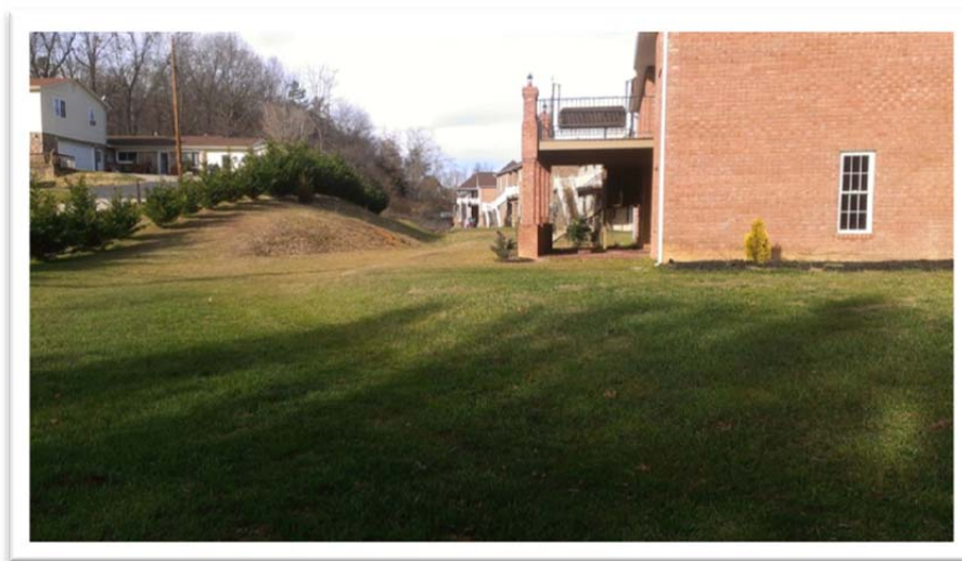
Figure 9: Channel behind homes along Cumberland Drive (looking US)
