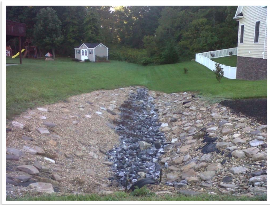
Figure 10: Upstream extent of Project Reach – Baybrook Drive inlet (looking US)
