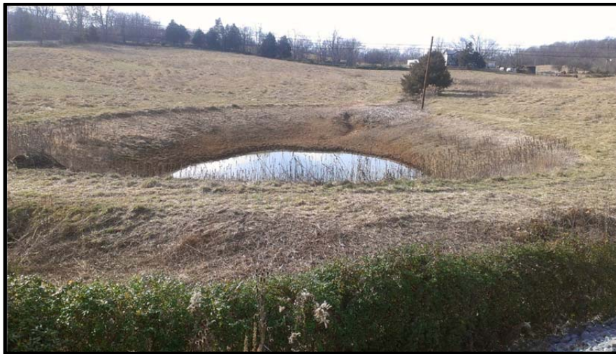
Figure 19: Port Republic – Spaders Church Rd Site, looking west from Port Republic Rd.
