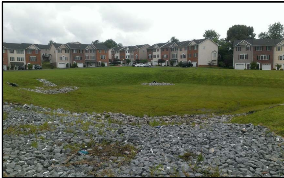
Figure21: Taylor Springs Site, looking northwest
